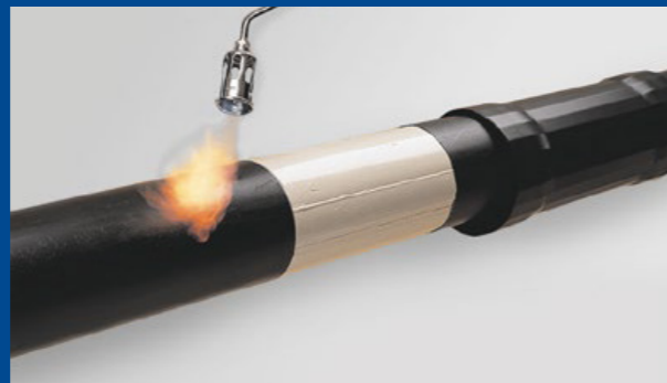
Assembly of insulation half shells
